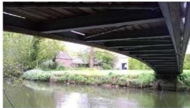
Figure 11: Footbridge over river
